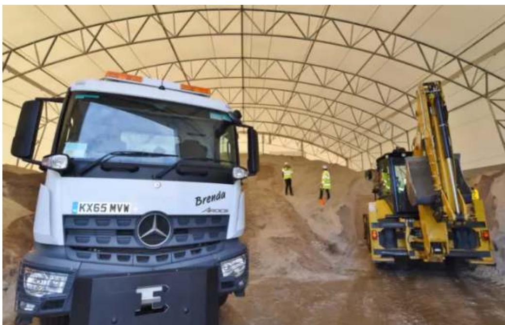
New Salt Barn at Highways Depot
