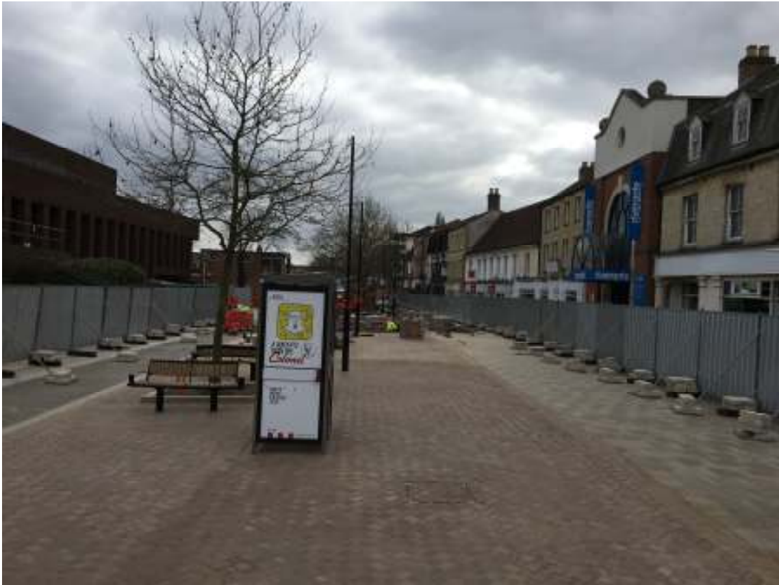
Lower Bridge Street Improvements
