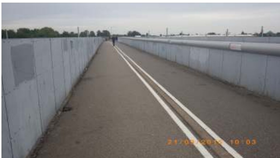
Westwood Railway Footbridge - Before
